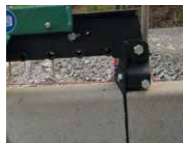
Precise Kerb Laying Special gripping jaw allows exact positioning of kerb
