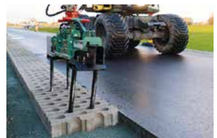
Working effectively Swing once for 4 layers and lay one after another
