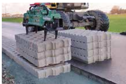
Installing first layer and picking up remaining three layers
