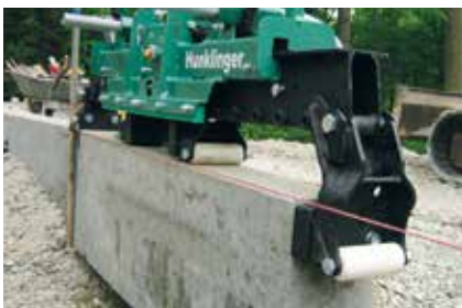
Lay against a guideline Exact lateral laying through long-sided grabbing
