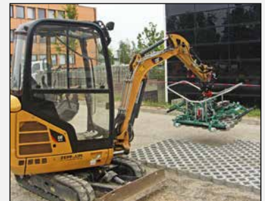
On small mini excavators cost-effective machine paver laying
