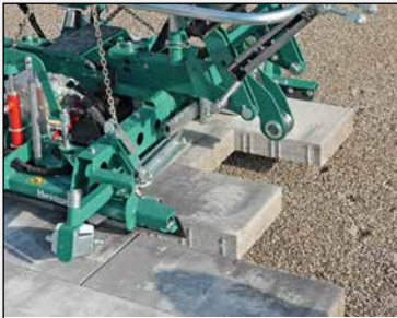
Large sized stones e.g. shift halfway and install 3 rows of 2 stones 60/30
