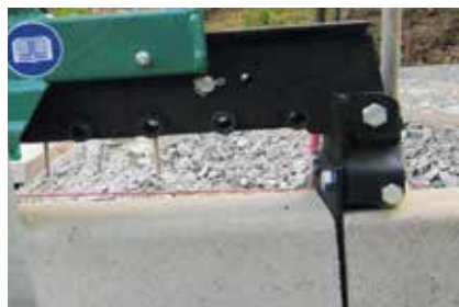
Precise kerb laying Special gripping jaw allows exact positioning of kerb
